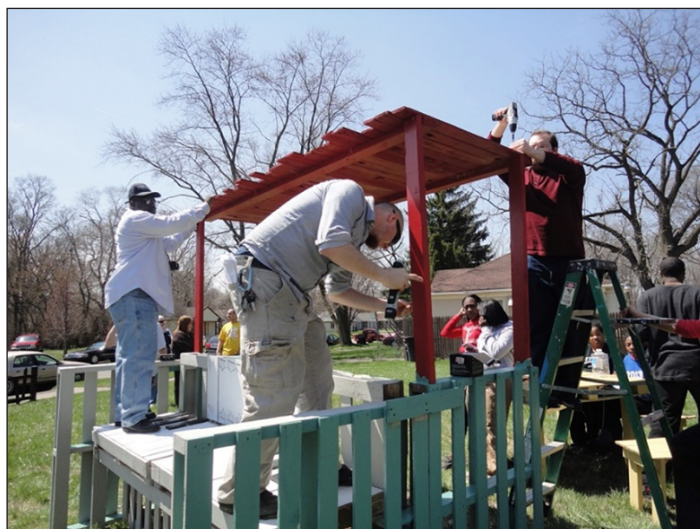
Figure 4 High school design-build work with Detroit Community Schools in Detroit.
